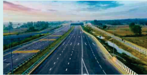
Expressway And Inter Connectivity Access
